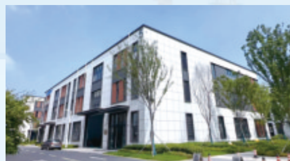
▲ TELFORD Changrong Factory
